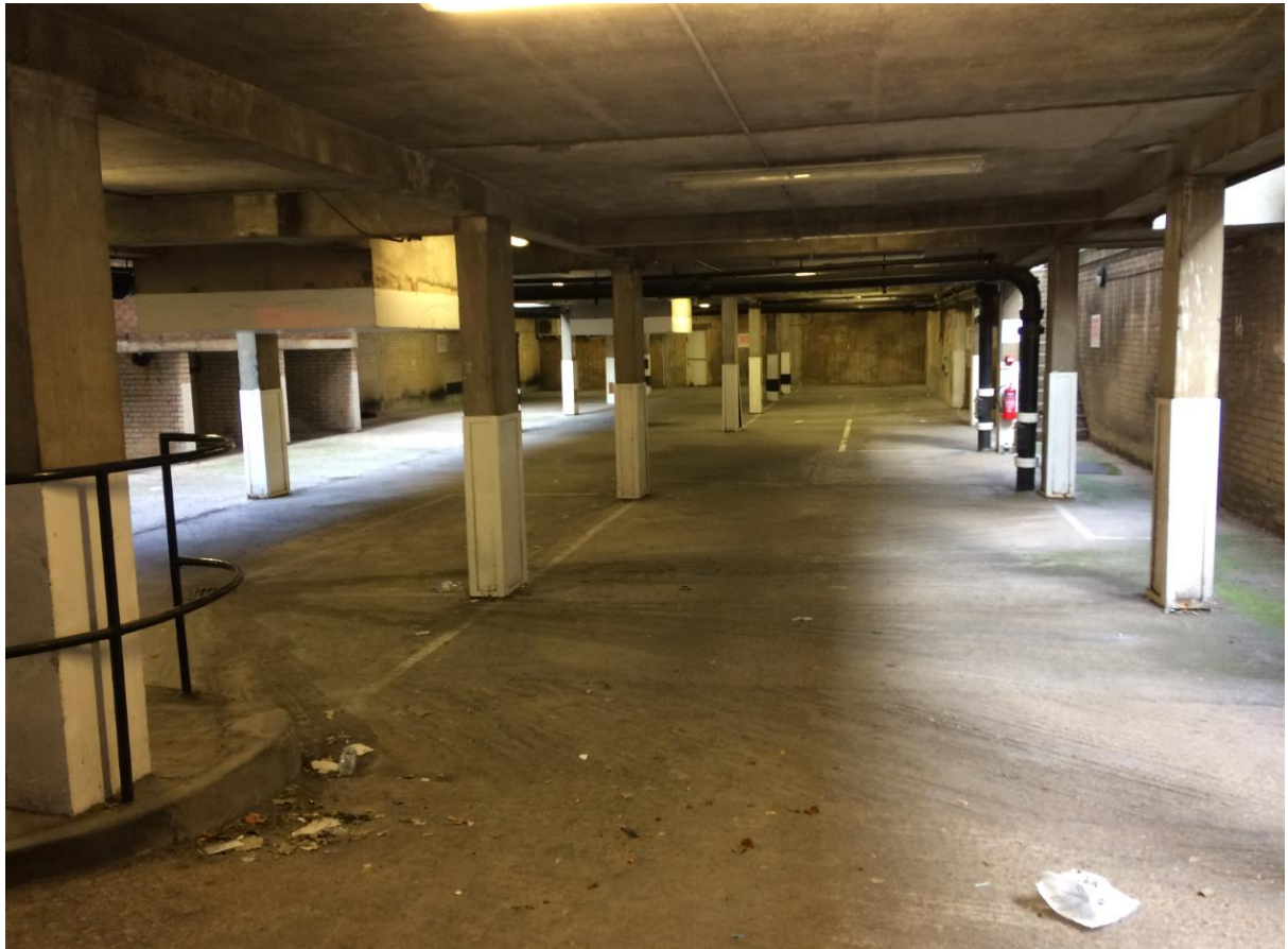
Internal car park:
